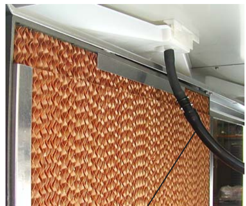
Hoses when fitted should not touch pads.
